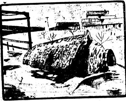
The cistern in the yard of Marion H. Church, Leon avenue, West Terre Haute, was floated from its foundation, ten feet below the surface, and toppied over on its side, when the water which broke through the Wabash river levee flooded the town. The cistern is of brick and concrete, ten feet deep and 71/2 feet in diameter. There was little water in the cistern at the time of the accident.
